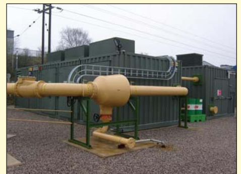
15" KSS Cyclone Separator Natural Gas Application
